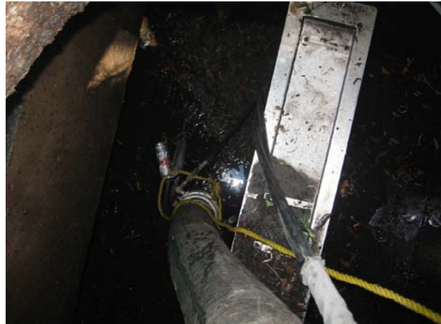
b. Standing water pumped from bottom chambers
