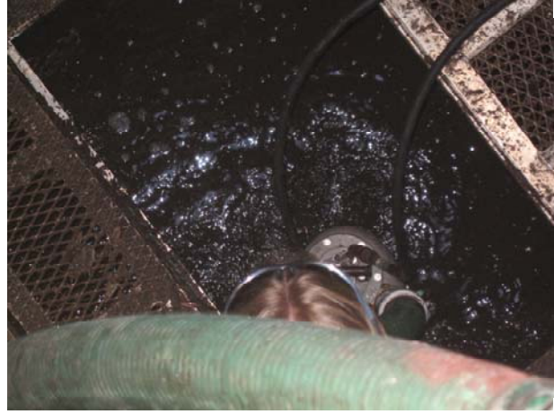
b. Water pumped from sump area
