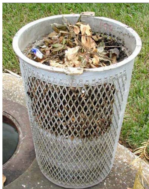
b. Basket filled with collected solids
