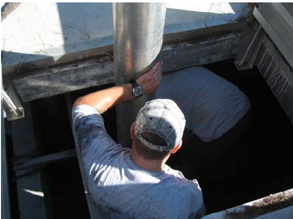
c. Solids removed from screen using vactor truck
