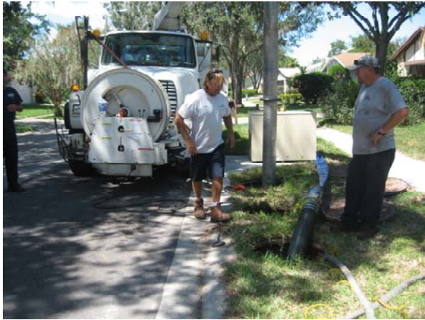
a. Clean-out operations
