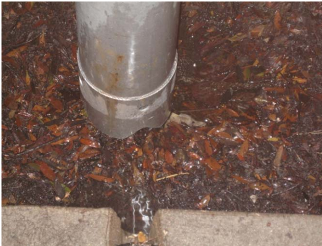
c. Solids removed from screen using vector truck
