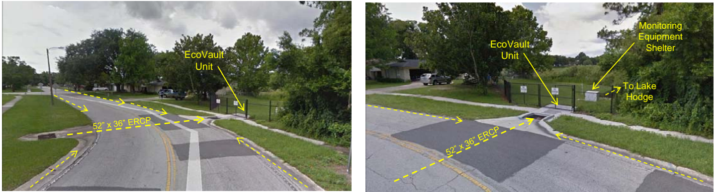
Figure 2-9. Photographs of the Lake Hodge Baffle Box Inflow.
