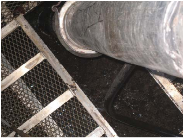
c. Solids removed using vacuum truck
