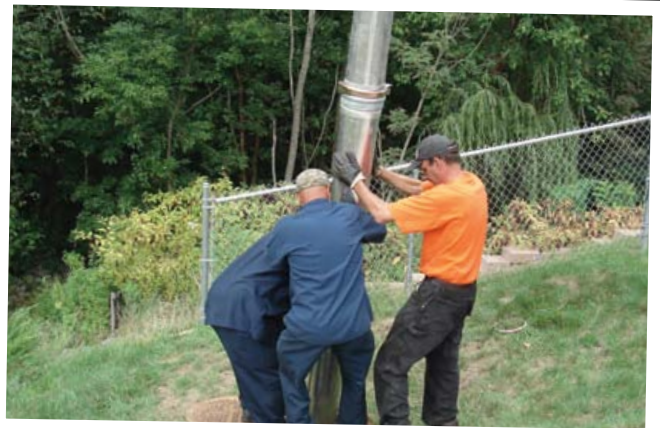
A vacuum truck excavates pollutants from the systems
