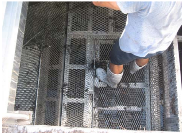
d. Screening following cleaning
