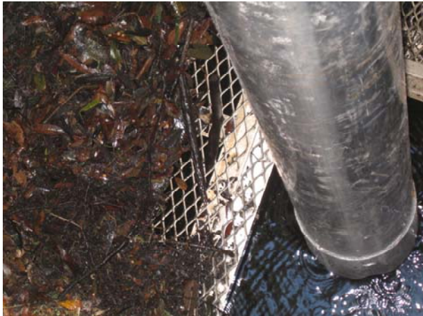
c. Solids vacuumed from chambers
