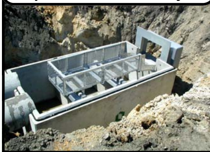
Step 3: Put sealant on joint
