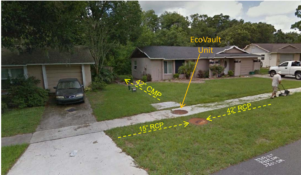
Figure 2-12. Photograph of the Exterior of the Gee Creek EcoVault® Unit.
