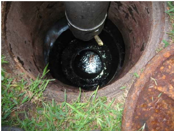
c. Sump area cleaned using vactor truck
