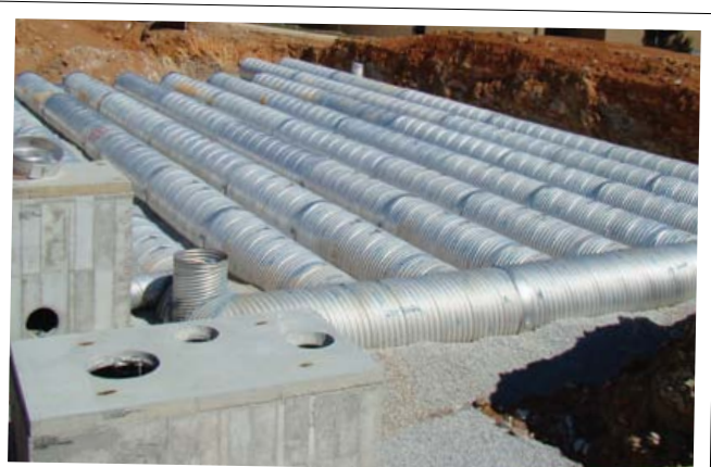
A Vortechs protects detention system from sediment build-up and reduces maintenance
