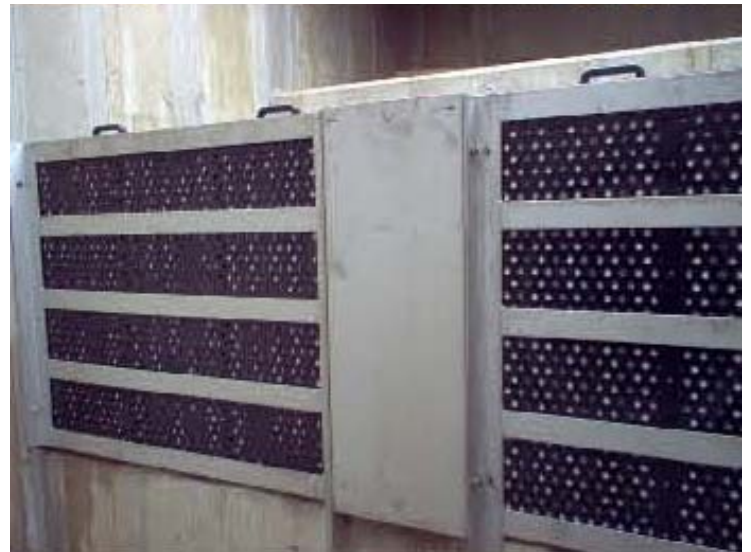
d. "Baffle Buddy" Outlet filter
