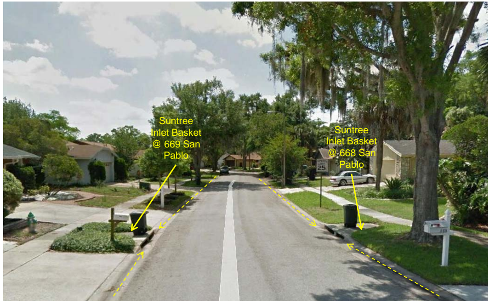
Figure 2-22. Photograph of the San Pablo Suntree Inlet Basket Site.
