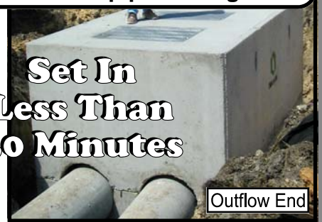
Ready to position inflow pipe and seal pipes with grout
