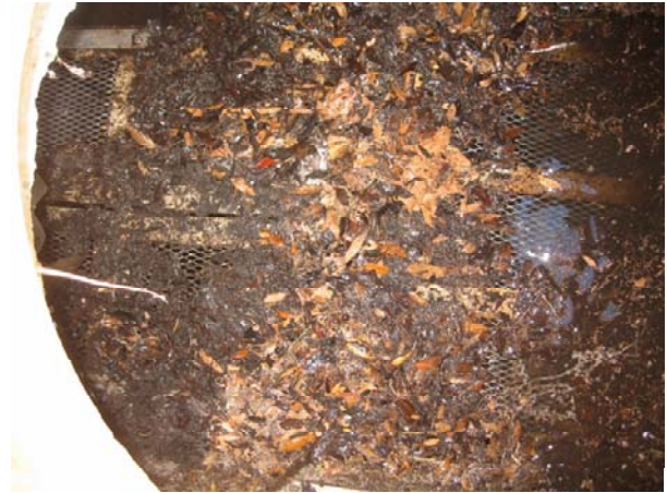
b. Vegetation screen prior to cleaning
