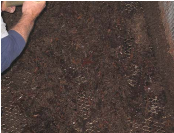
a. Accumulated vegetation on the screens
